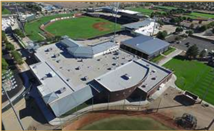
In 2015, the Royals Spring Training complex underwent an $8 million renovation, adding approximately 14,000-square feet.
